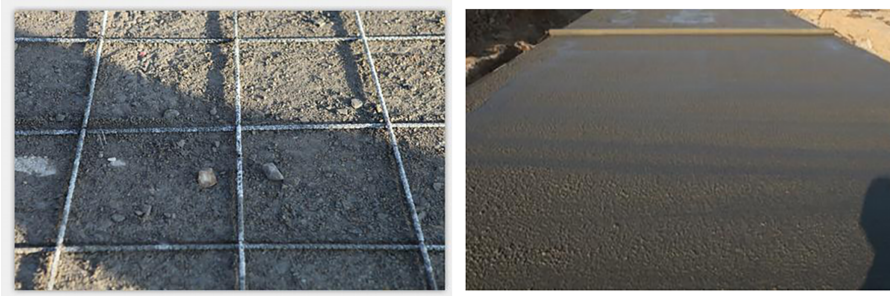
Figure 6: BF rebars for pavement.
