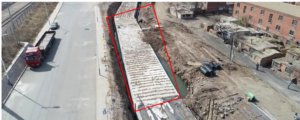
Figure 22: Underground culvert in a city.
