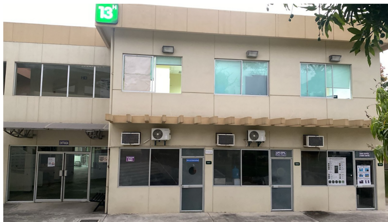
Figure 4: Exterior front view of building 13H at the Gustavo Galindo campus.
