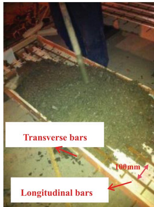
Figure 4: Longitudinal and Transverse bars
