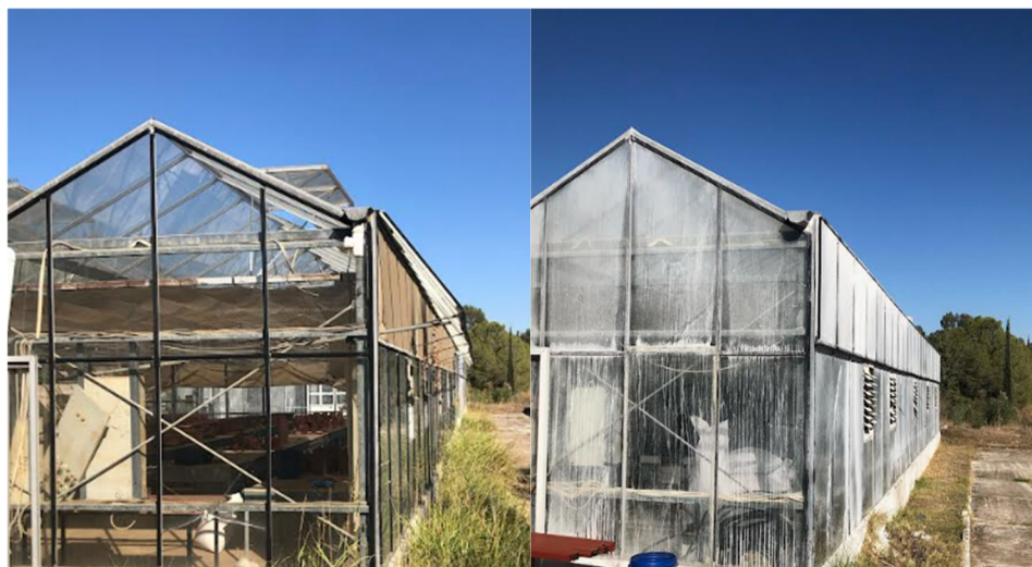
Figure 1: A greenhouse covered with lime to increase light reflection with air flow from a fan (on the right), and a greenhouse without ventilation and without lime-covered windows (on the left).
