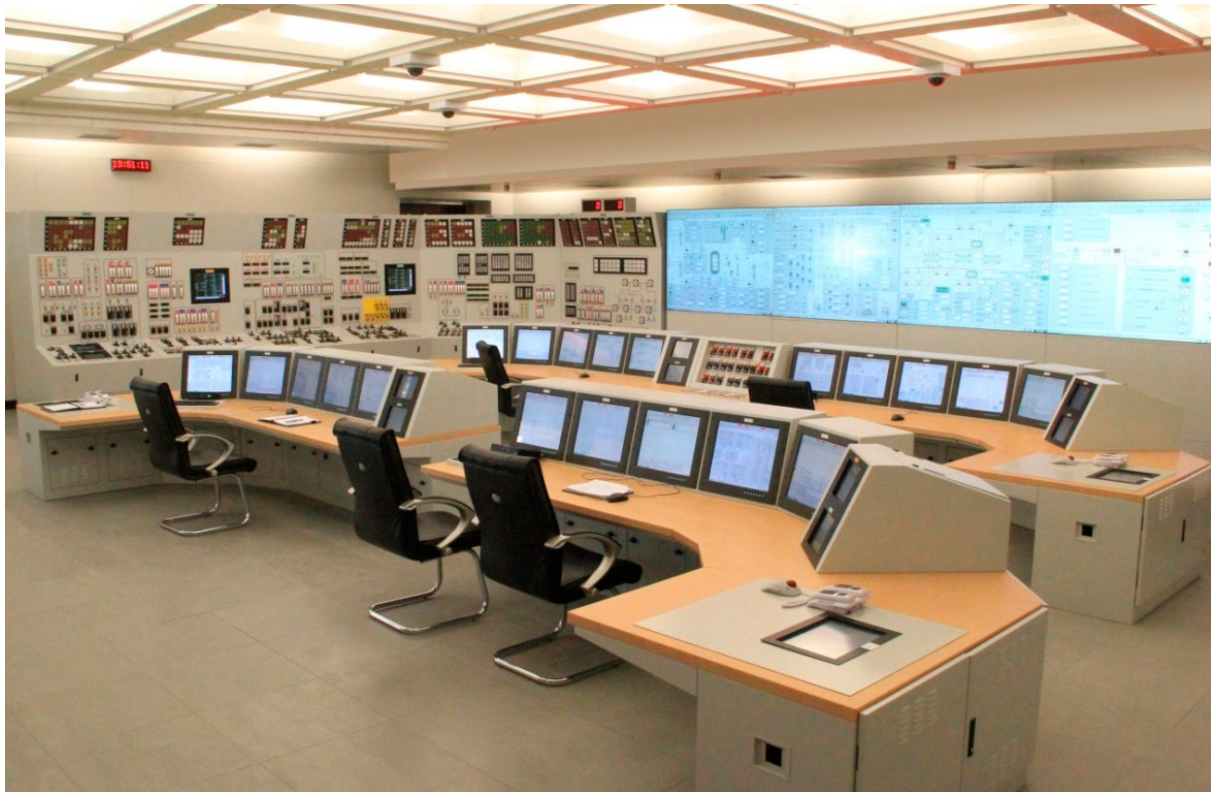
Figure 1: Photograph of the full-scope verification simulator.
