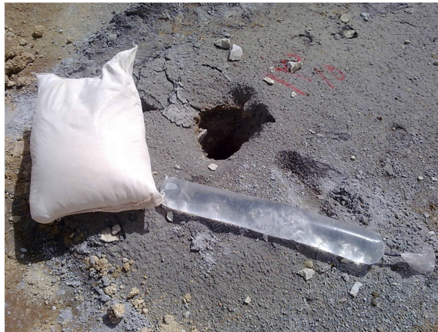
Figure 21: Ionized water ampoules and blasting hole (based on Abdollahisharif et al. [22]).
