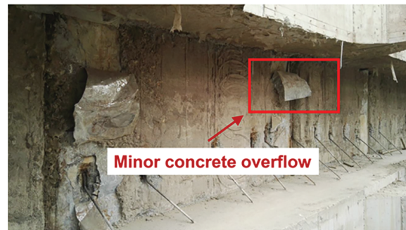
Figure 1: Concrete extrusion caused by local instability (Sanyang Road, Wuhan, China)
